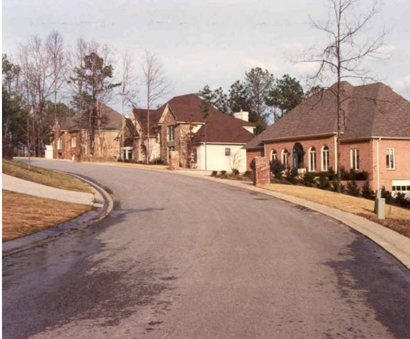
Figure 4. Example of Site General View
